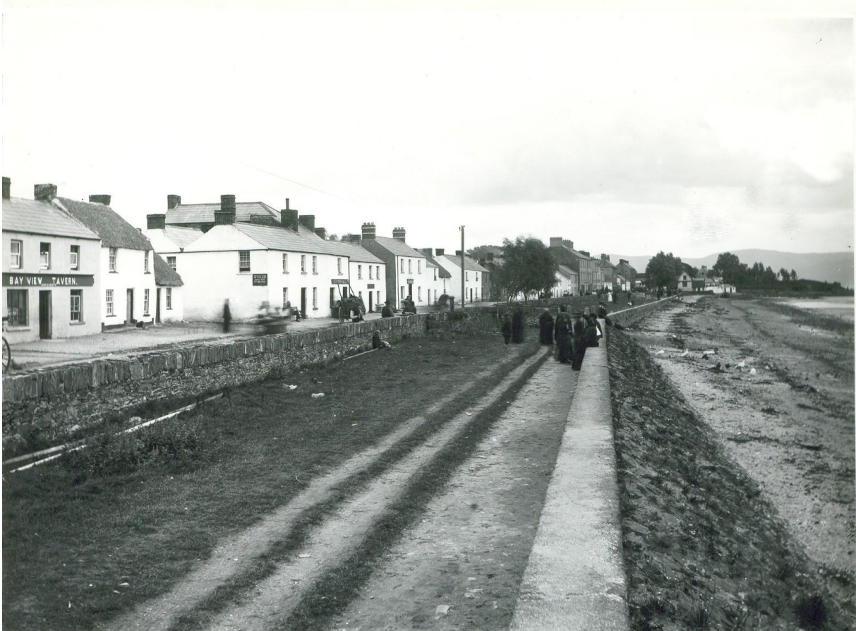
Photo 1: Beach and promenade circa 1890. Note band of dry sand below sea wall.
