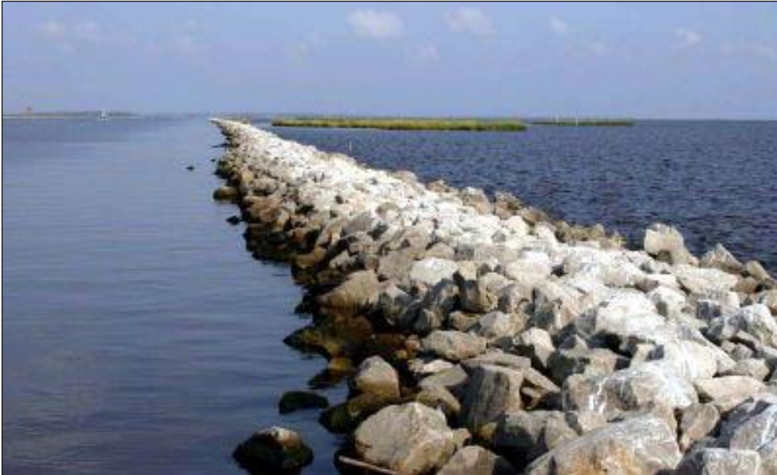
Figure 2-9: Example of a rock wave barrier
